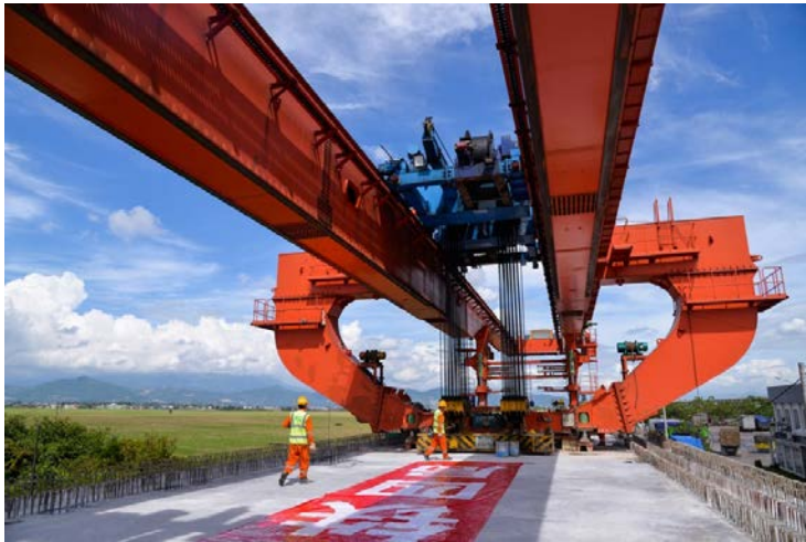
Picture 2: Girder Launcher in Jakarta-Bandung Speed Train Project Source
