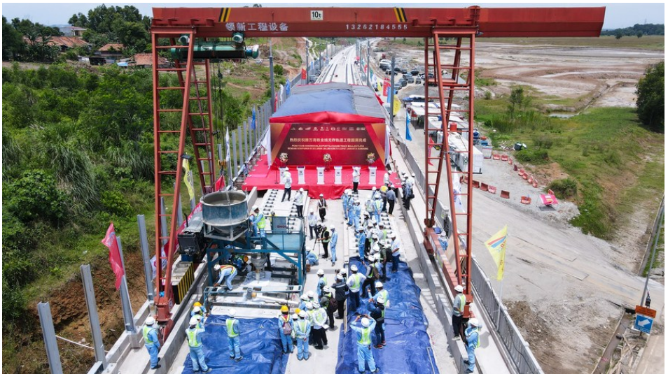
Picture 4: Installation of Ballastless Track
